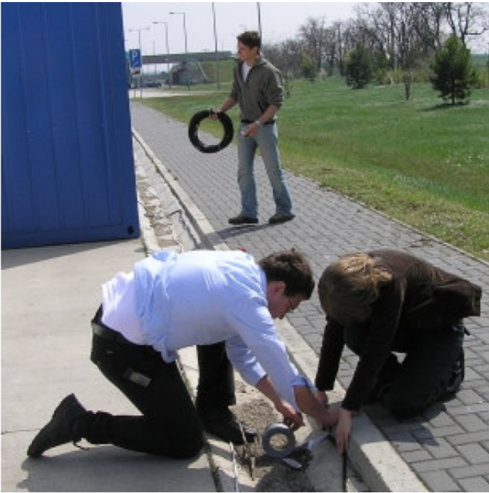
Quantum mechanics at work: Installing an optical quantum channel at the Austrian-Croatian border, 2005
